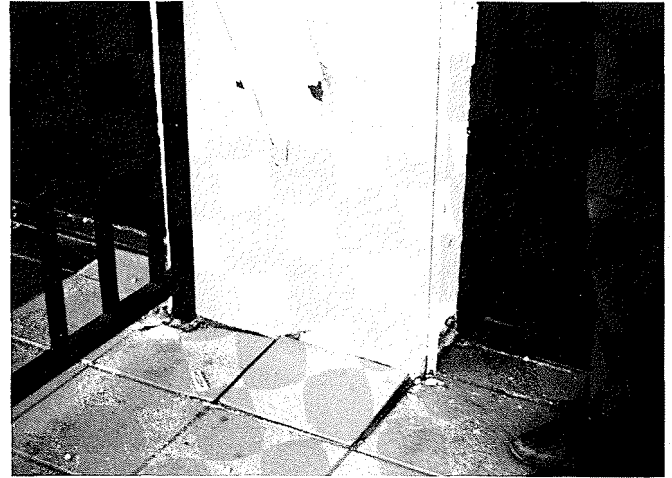
Fig. 6. First Interstate Bank Building in Northridge: column uplift at the base of the X-bracing.
